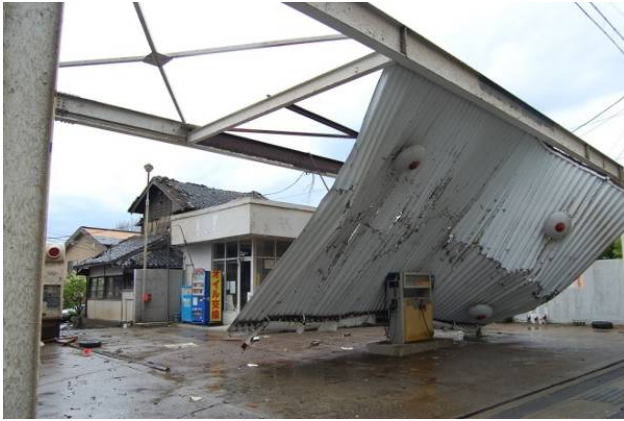
Photo 30 Collapse of a gas station roof Photo 31 Heavy deformation of roof of a bicycle park
