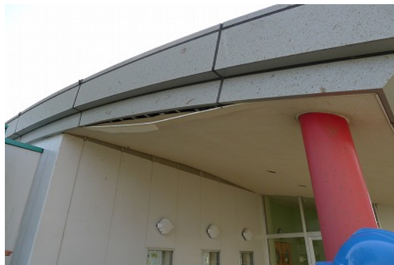
Photo 40 Breakage of exterior and windows Photo 41 Breakage of eave soffits
