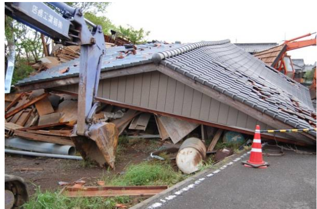
Photo 4 Wooden Building C
