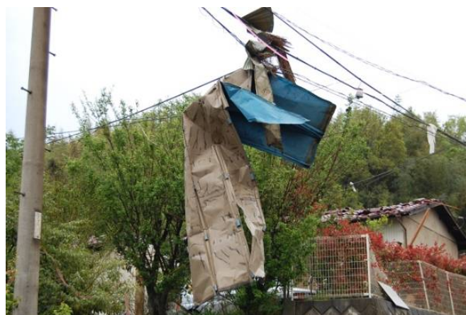
Photo 29 Roofing materials hung at electric cables
