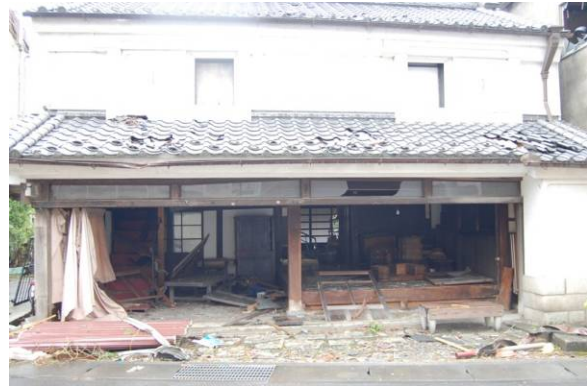
Photo 14 Wooden Building L
