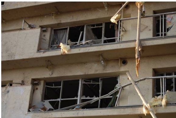
Photo 22 Windows and handrails 1
