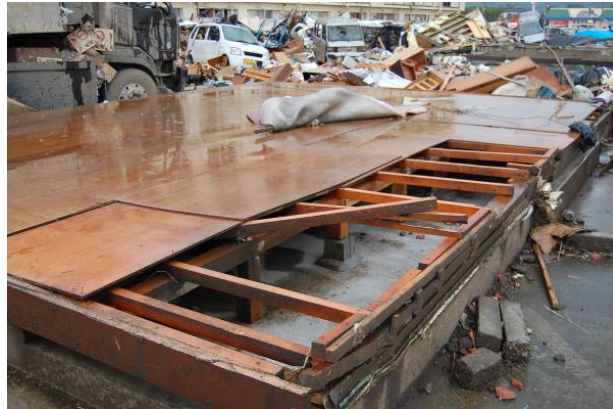
Photo 7 Wooden Building E
