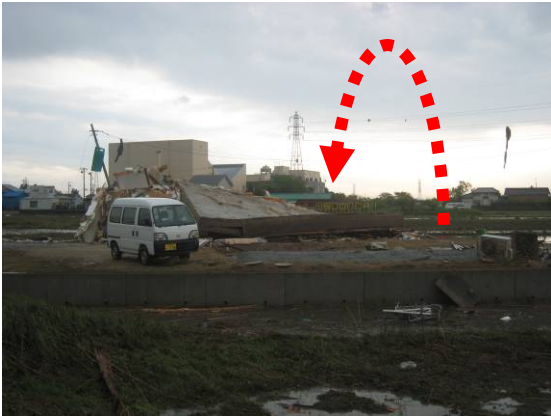
Photo 1 Wooden Building A
