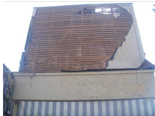
Photo 16 Wooden Building N
