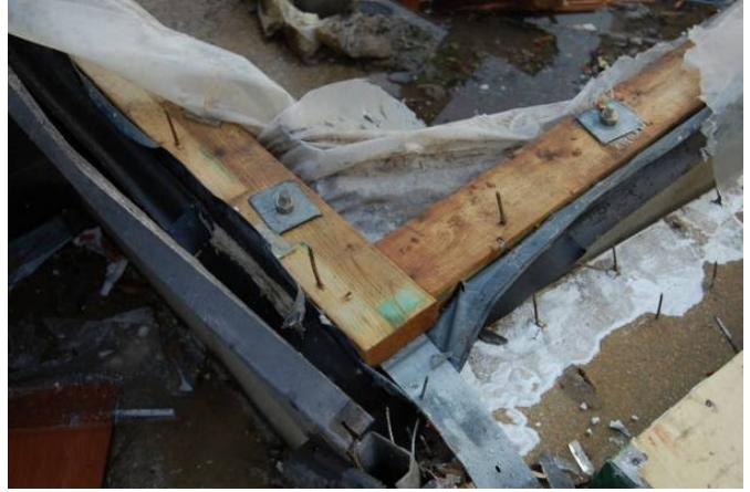
Photo 5 Wooden Building D Photo 6 Remaining foundation beam of Wooden Building D
