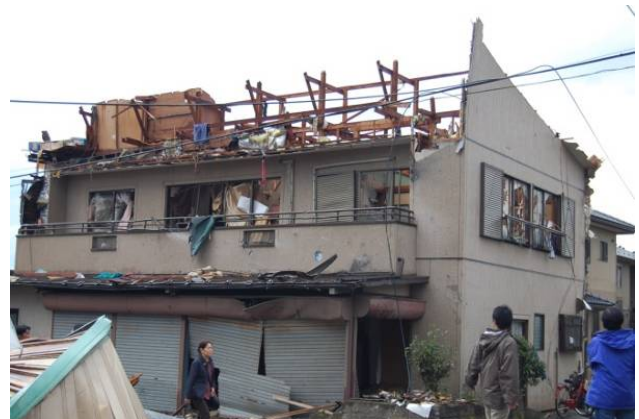
Photo 12 Wooden Building J
