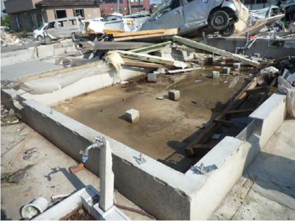
Photo 5 Wooden Building D Photo 6 Remaining foundation beam of Wooden Building D
