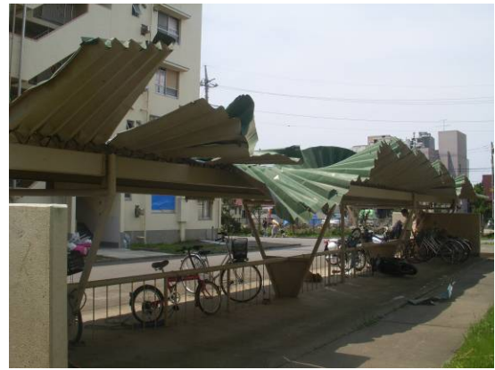
Photo 30 Collapse of a gas station roof Photo 31 Heavy deformation of roof of a bicycle park
