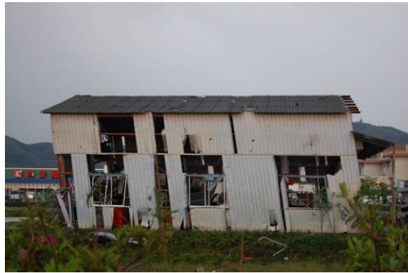
Photo 18 Steel Framed Building B
