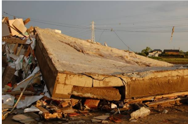
Photo 2 Turned flat basement of Wooden Building A
