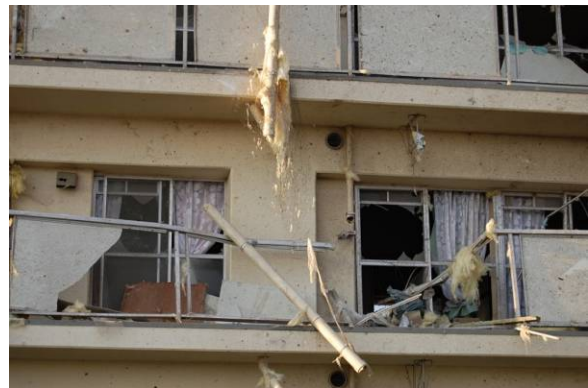
Photo 23 Windows and handrails 2
