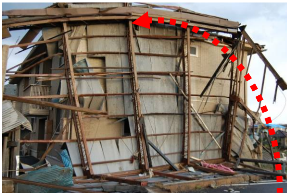
Photo 19 Steel Framed Building C
