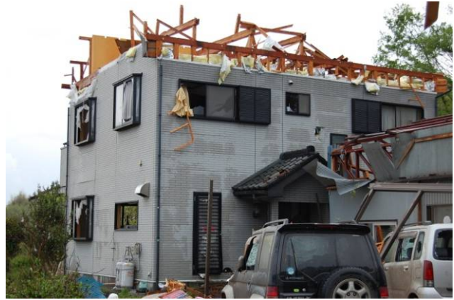
Photo 10 Wooden Building H
