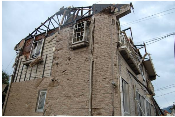
Photo17 Steel Framed Building A
