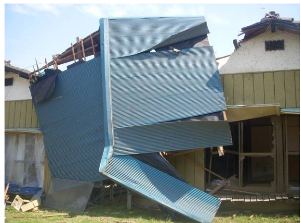
Photo 28 Collision of flying roof frame
