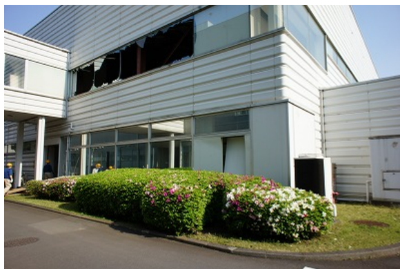
Photo 38 Broken window of a roofed passage Photo 39 Broken window of exterior wall
