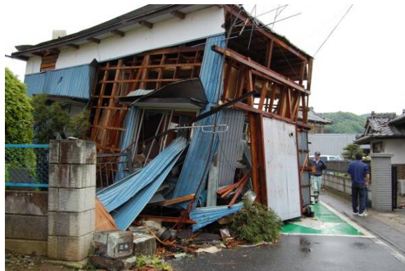
Photo 8 Wooden Building F
