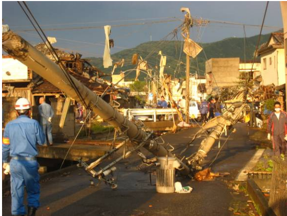
Photo 33 Broken / inclined electricity poles 1
